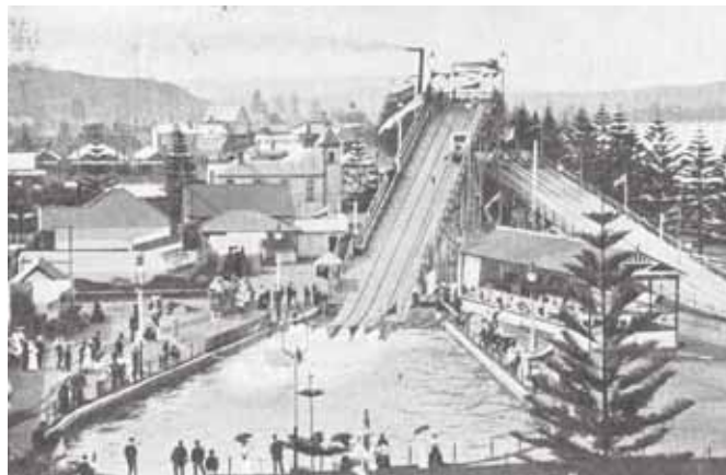
Manly Water Chute built 1903 - was on the cnr of South Steyne and Ashburner Street. It had originally been Joseph Smith's dairy farm, with a frontage to the creek where the surf club now stands. For many years this site was used for 'resort' style attractions, including Manly's first cinema, later a roller skating rink, then the site of Dungowan's cabaret/ice skating rink.
