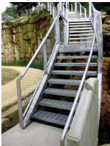
New steps from Waverton Park entry to top terrace level. Source: Simon Wood photography
