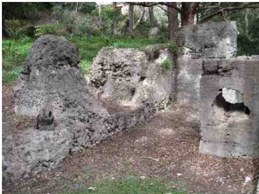
Old infrastructure of John W. Eaton Ltd, timber merchants, at Sawmillers Reserve
