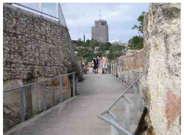
BP Site, stone gabions and cut sandstone along the paths
