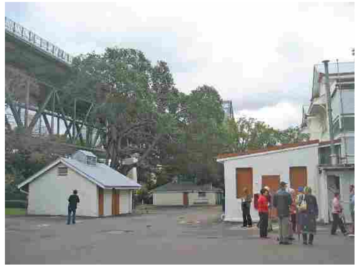
View of the Story Bridge from the rear of Yungaba
