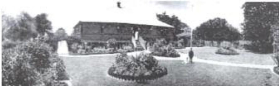
Mornington Charters Towers 1917
