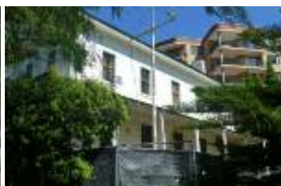
Cleveland House, Surry Hills with only trees for privacy from overlooking
