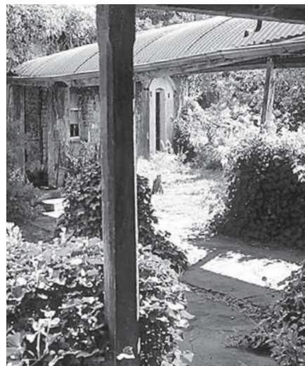
Covered walkway at rear of house.
