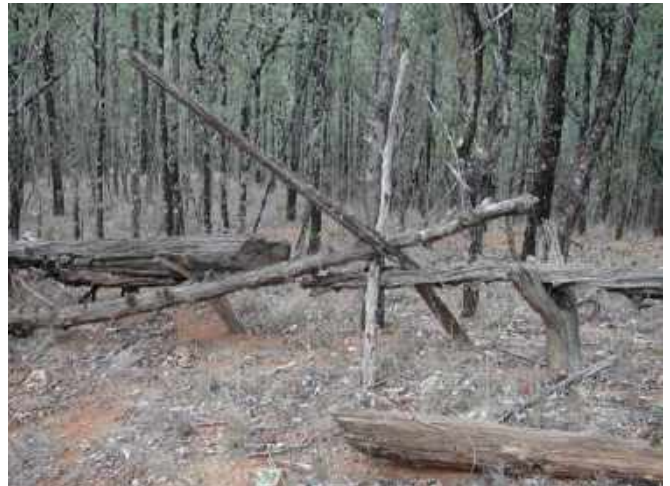
Dog-leg fence with logs resting on forked posts, Mt Trooper, NSW.
