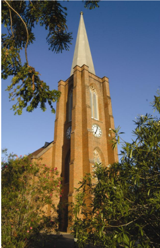
St John's Church, Camden
